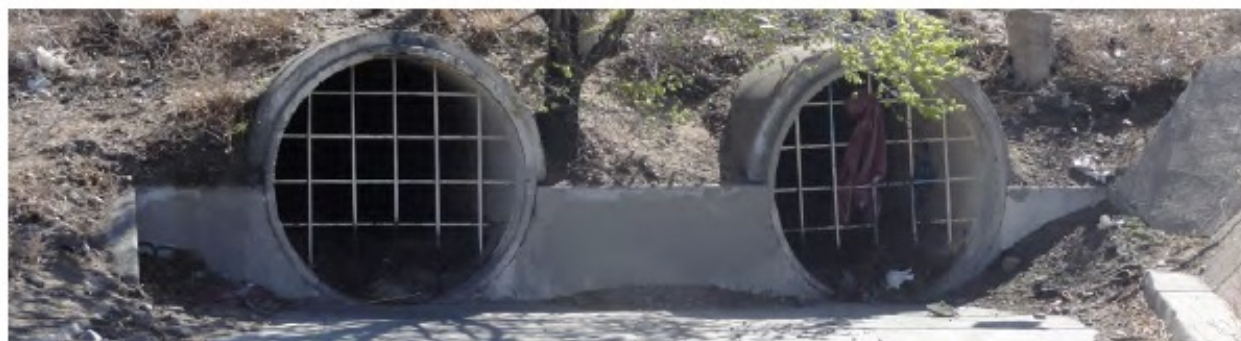
Culvert under Interstate 25, Albuquerque, NM (photo by Tess Houle)
