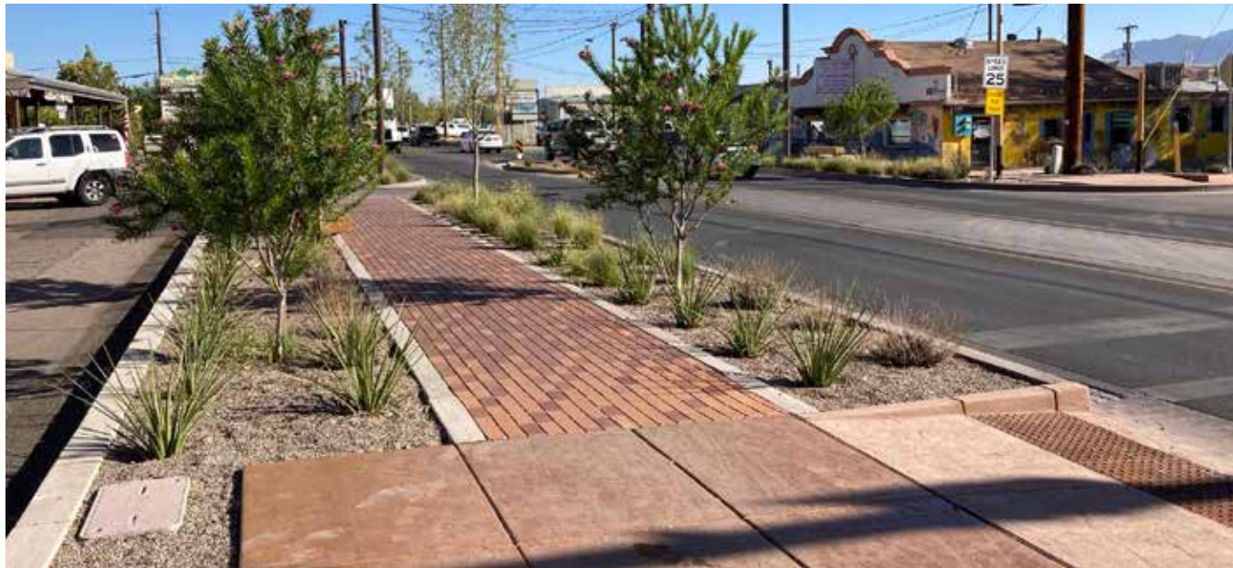
4th Street permeable pavers, Photo by Sites SW
