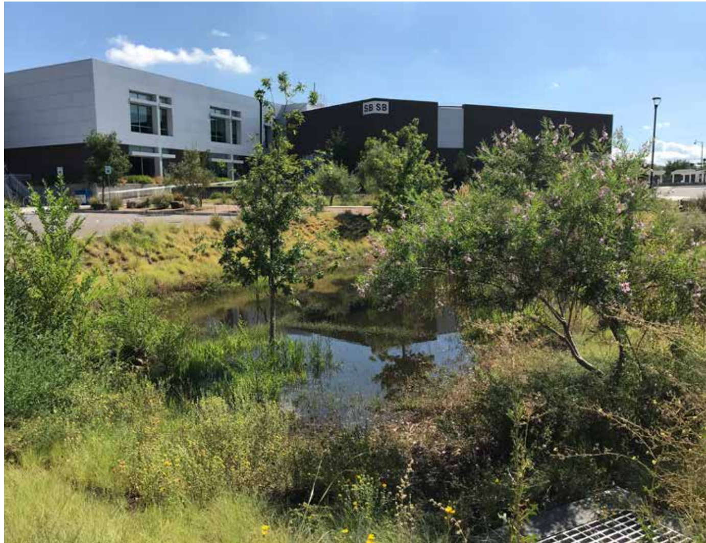
Runoff captured in stormwater harvesting basin at CNM
