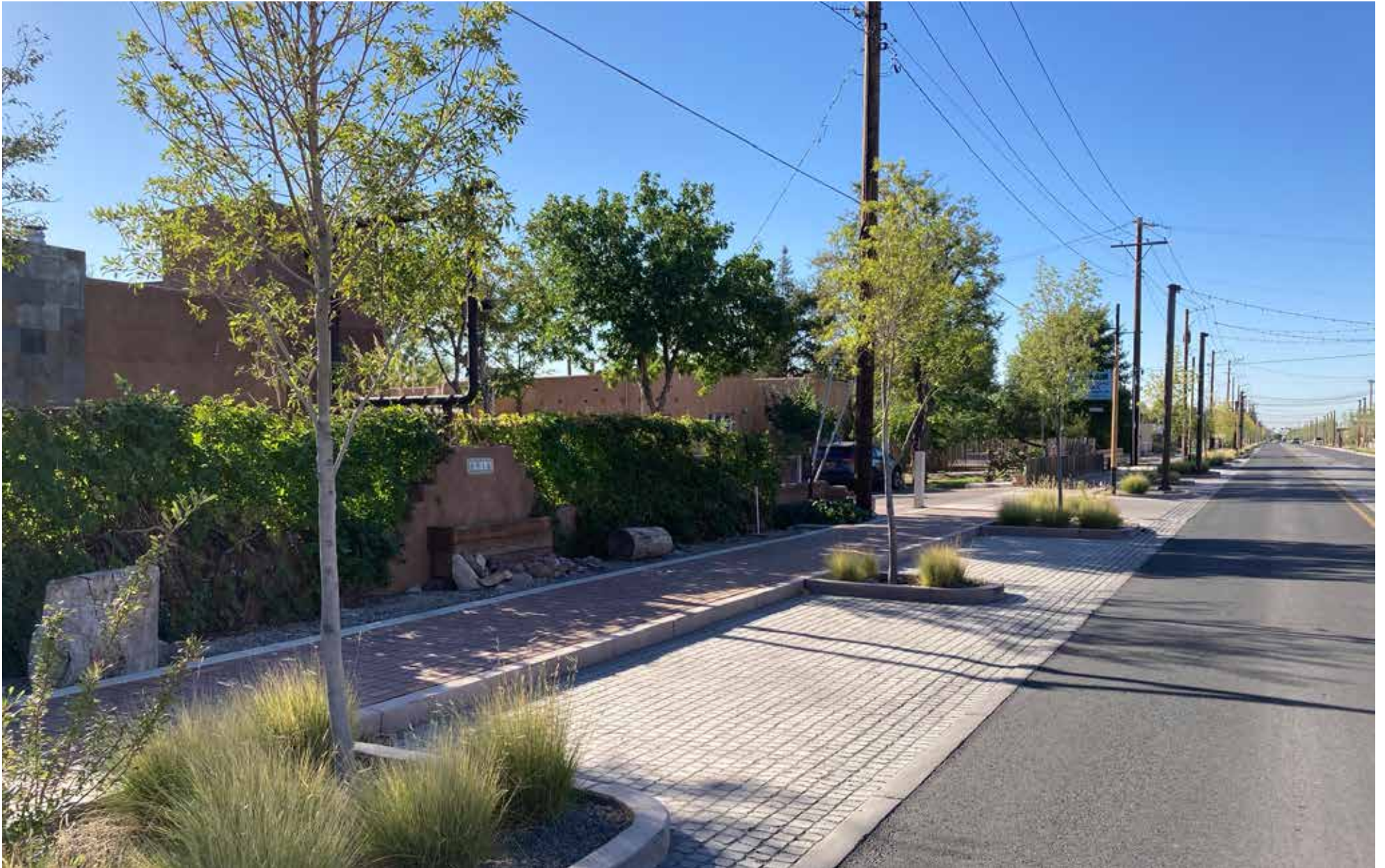
4th Street Permeable Pavers, Photo by Sites SW
