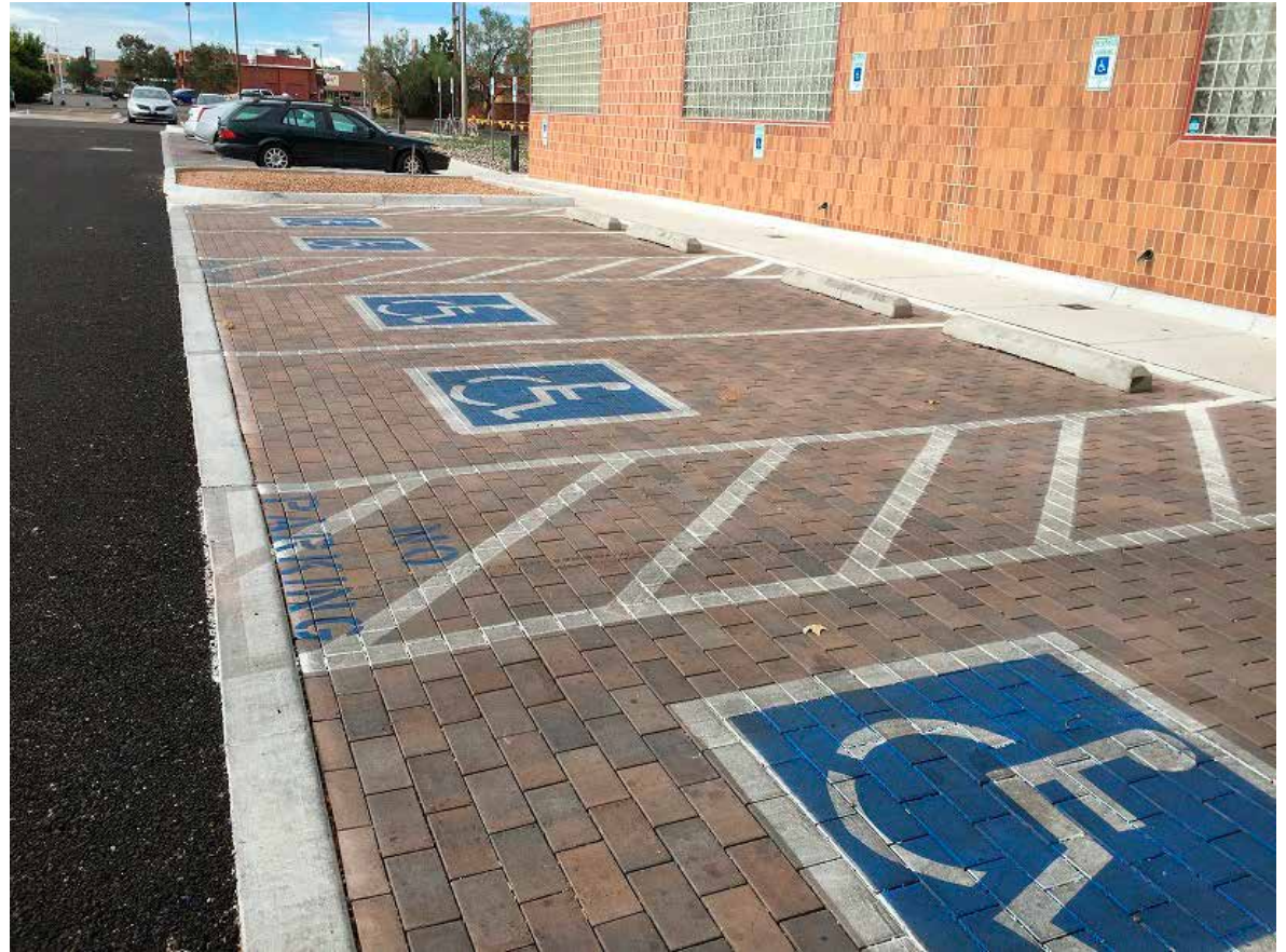
Wheelchair accessible permeable pavement
