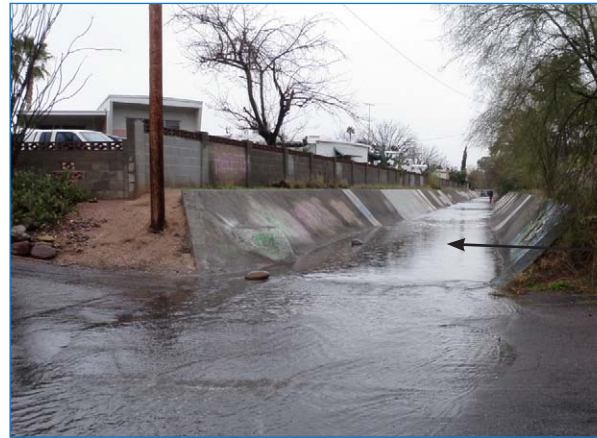
Grey infrastructure: a concrete channel sends stormwater quickly downstream.
