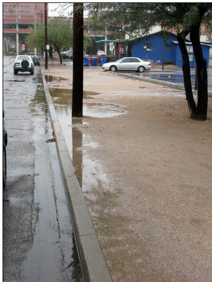
Before: At this University of Arizona parking lot, small curb cuts allowed stormwater to flow past existing trees onto the pedestrian area in the ROW, and then on to the street.
