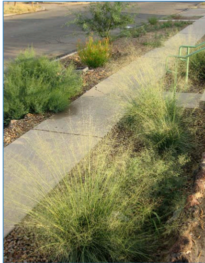
Native bunch grasses (foreground) thrive in a swale that collects stormwater runoff from a parking lot (right, not shown).
