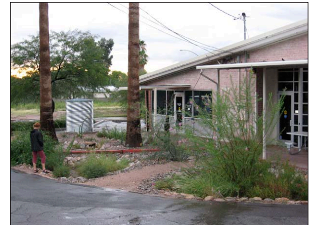
One year later, stormwater-fed native vegetation grows to soften the offices' stark facade and shade an outdoor patio. Note that basin slopes are lined with rock to reduce erosion.
