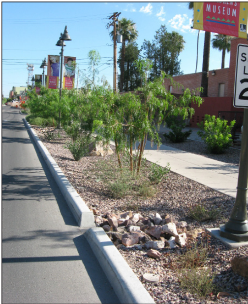
This long, shallow ROW swale has multiple curb cuts along its length.
