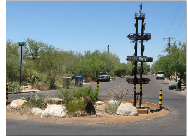
At the top of its sub-watershed, this traffic circle (right) was designed to capture and retain the rain that falls on it.
