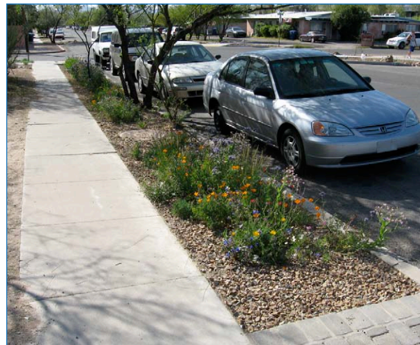
At this site in Tucson, a 3" deep swale was created in the ROW to collect runoff from the sidewalk and adjacent property.
