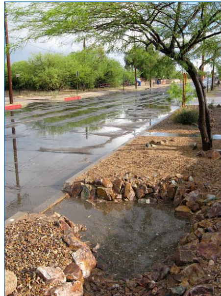
Green infrastructure: a curb cut captures stormwater from the street to feed vegetation.
