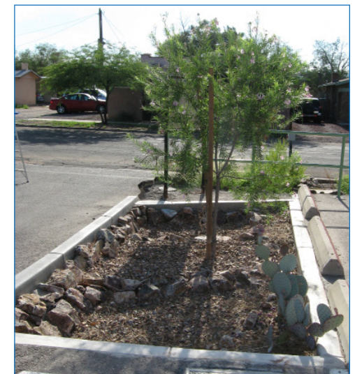
At this University of Arizona parking lot, an unused space happened to coincide with the lot's natural low point. The asphalt was removed and a bioretention basin installed. Note concrete header and curb stops. The basin's interior was terraced and shaped to distribute stormwater evenly. Overflow exits the back left corner to the street.
