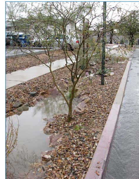
A velvet mesquite tree is planted on a terrace above the level of stormwater inundation at this GI site.
